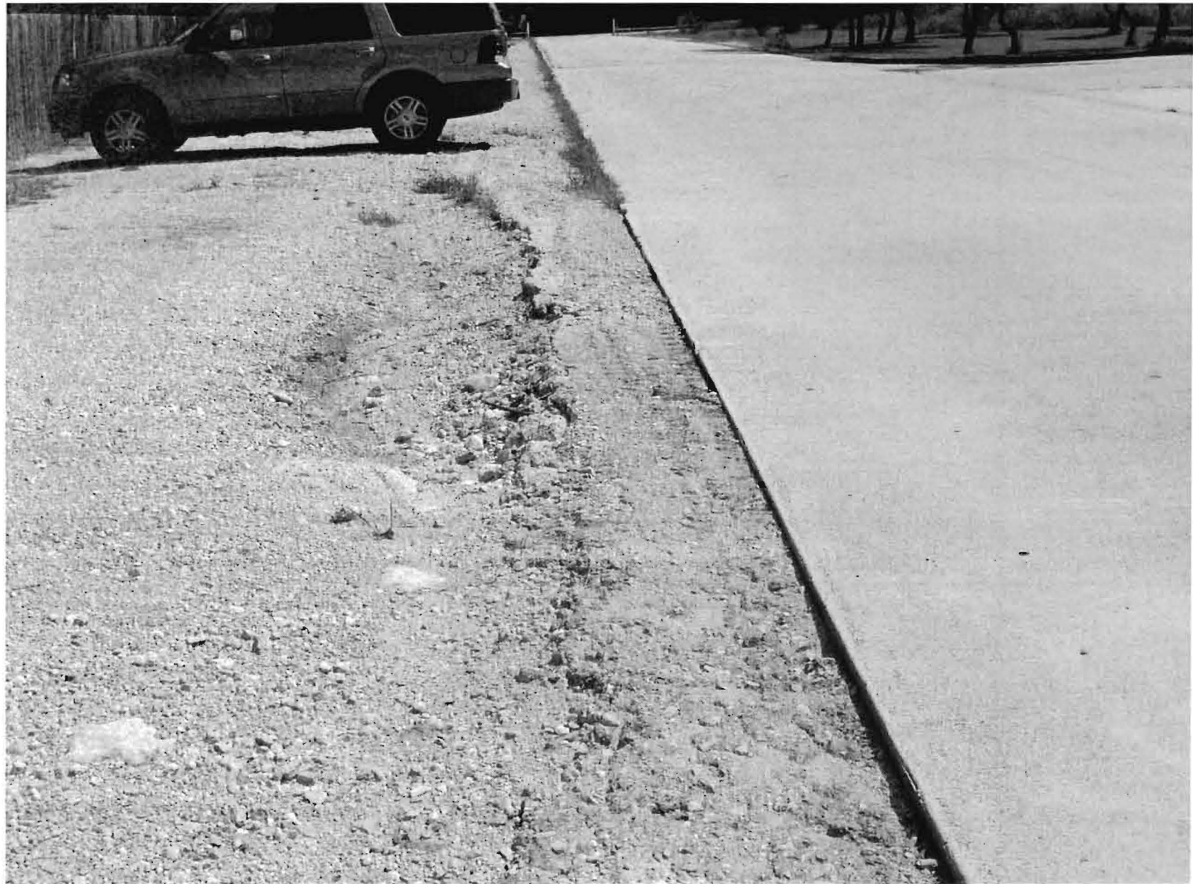
Arlon Seay Elementary School — Erosion on Existing Compacted Base Area in Front of School
