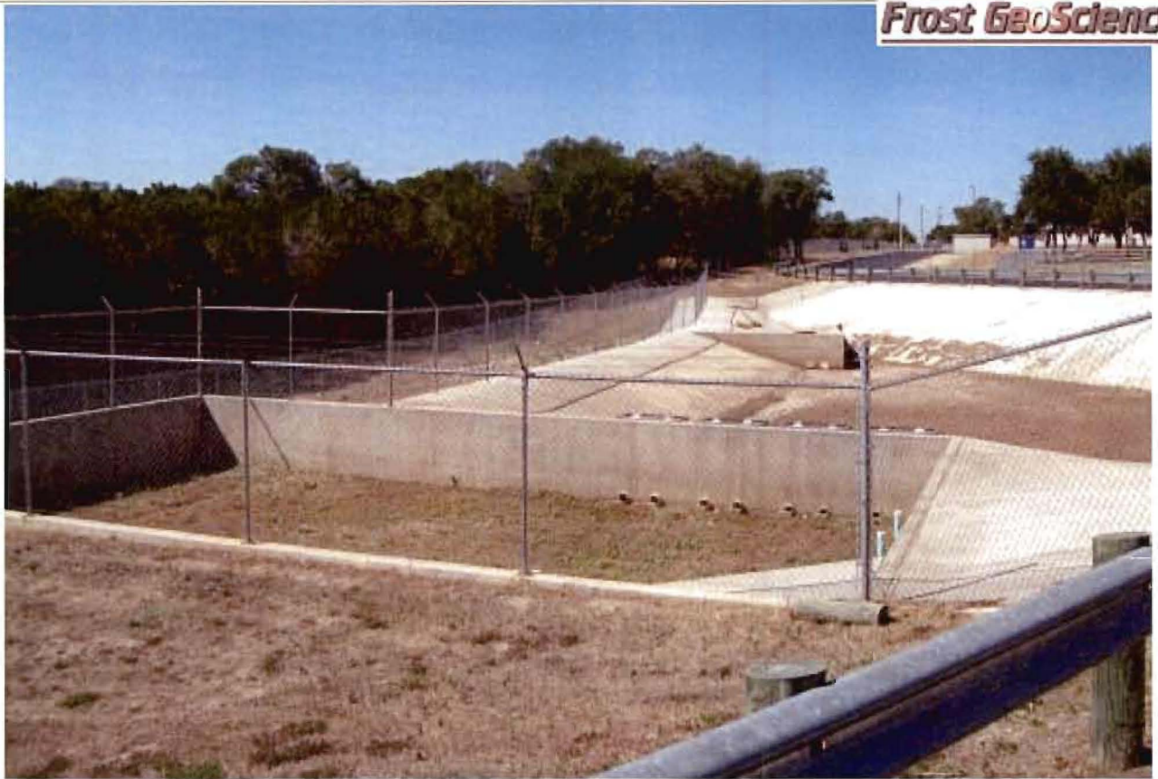
View of a stormwater basin and sand filtration basin in Area 2.
