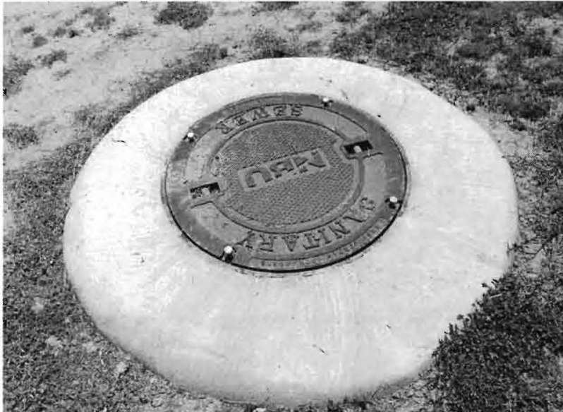
Photo #3 View of sanitary sewer manhole typical of features F-2 and F-4.
