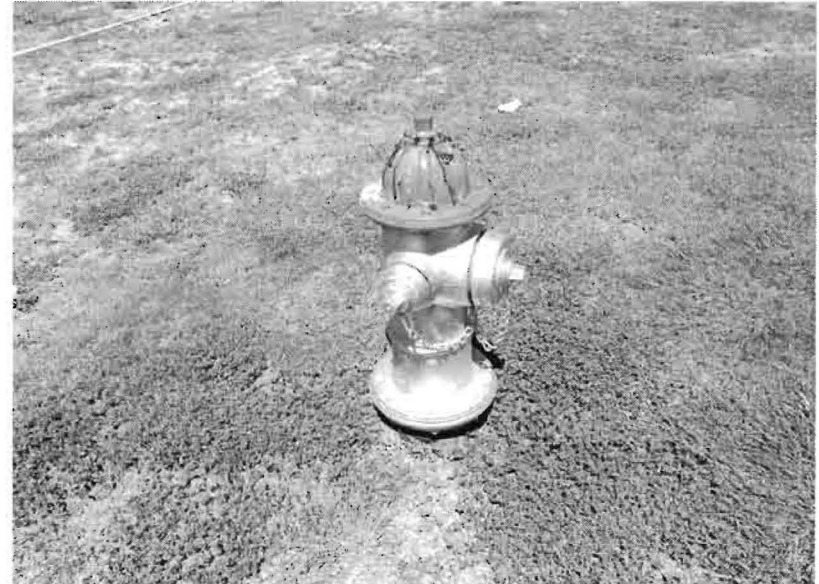
Photo #4 View of fire hydrant (feature F-3).
