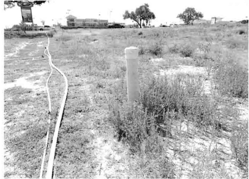
Photo #2 View of sanitary sewer stub-out typical of features F-1, F-5, F-6, and F-7.
