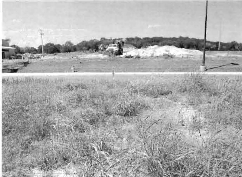
Photo #5 View of utility trench along the western property line demarcated by a gas placard.
