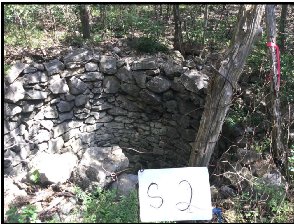
S-2: Old rock-lined, hand-dug well.
