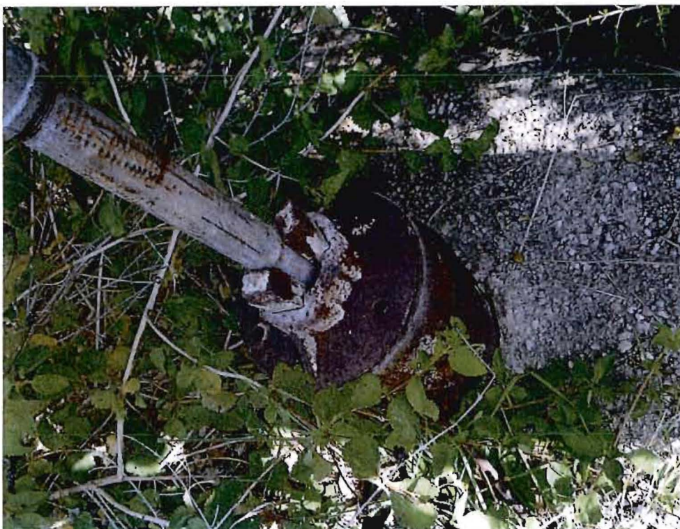
S-10: water well with separated casing, sensitive
