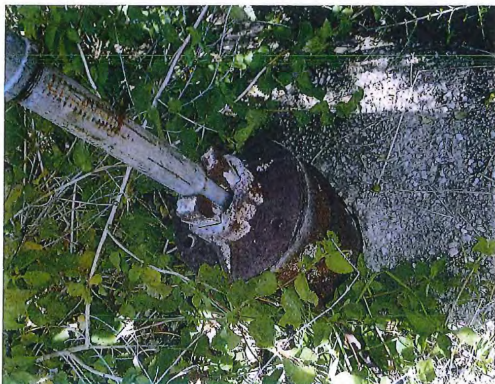
S-10: water well with separated casing, sensitive
