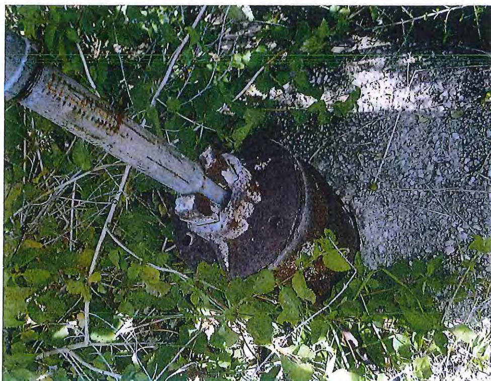
S-10: water well with separated casing, sensitive
