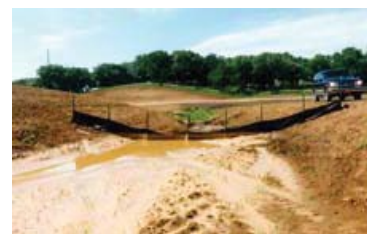
Figure 8. Proper installation, bottom of both ends are above the top of the middle.
