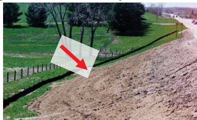
Figure 4. Avoid long runs of silt fence
