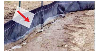
Figure 16. Poor compaction has resulted in infiltration and water flowing under this silt fence causing retained sediment washout.
