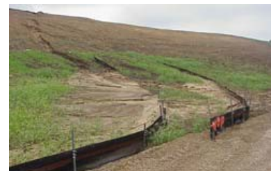
Figure 23. New silt fence below the old fence
