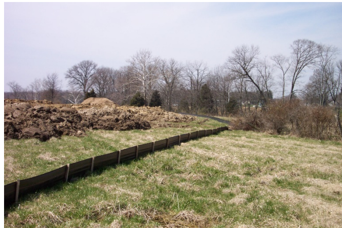
Figure 1. A silt fence at the perimeter of a construction site.
