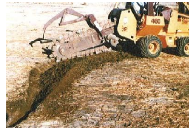
Figure 15. Trenchers make a wider excavation at turns.
