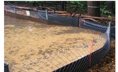
Figure 11. Chain link supported silt fence
