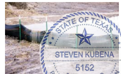
Figure 3. Water flowing over the filter fabric during a rain event.
