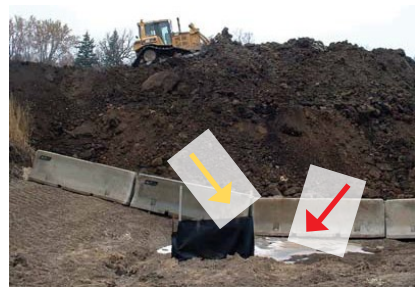
Figure 18. Front of silt fence on part of stockpile's perimeter.
