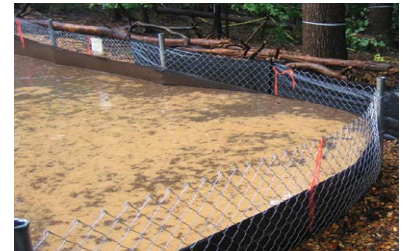
Figure 11. Chain link supported silt fence
