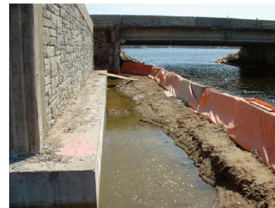
Figure 19. Silt fence for bridge abutment excavation.
