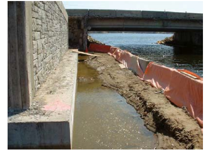
Figure 19. Silt fence for bridge abutment excavation.
