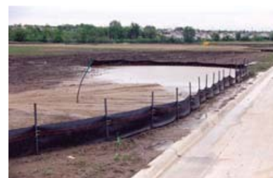
Figure 10. Gentle slopes may require a silt fence
