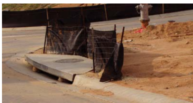
Figure 7. This silt fence doesn't work
