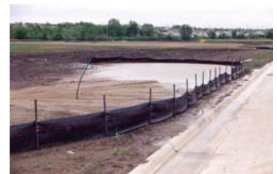
Figure 10. Gentle slopes may require a silt fence
