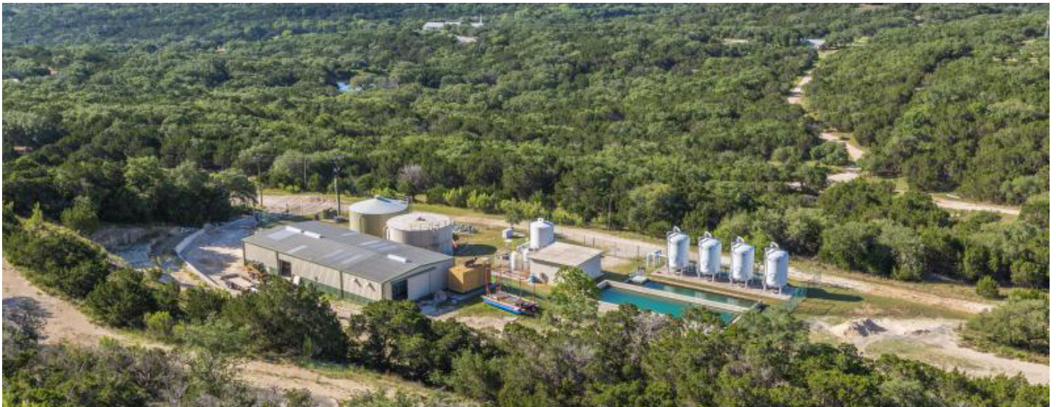
Wastewater treatment Facility at Old Triple Peak Drive, south of Canyon Lake (facing south)
