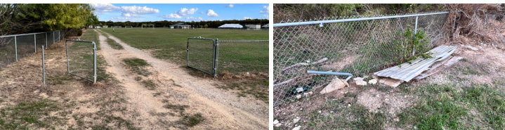
The fence line at the soccer field parking lot requires immediate repair. The shade structure and playground surfacing require immediate replacement due to safety concerns and potentially falling debris.
