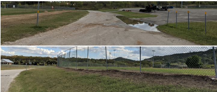
Park drive grading causes water to pool in many locations. Park drive and fence edging are often muddy and require reseeding. Minor fence repairs are needed at the central diamond field and football field.
