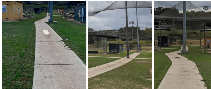
Sidewalks along many diamond fields are obstructed by utility and light poles, requiring re-alignment and repair of depressions and cracking along edges.
